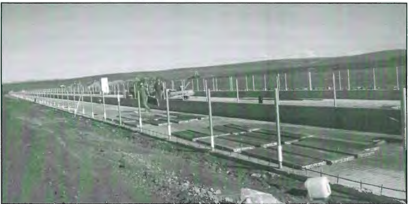
Construction of Chris Drew's Feed Pad at Burra
