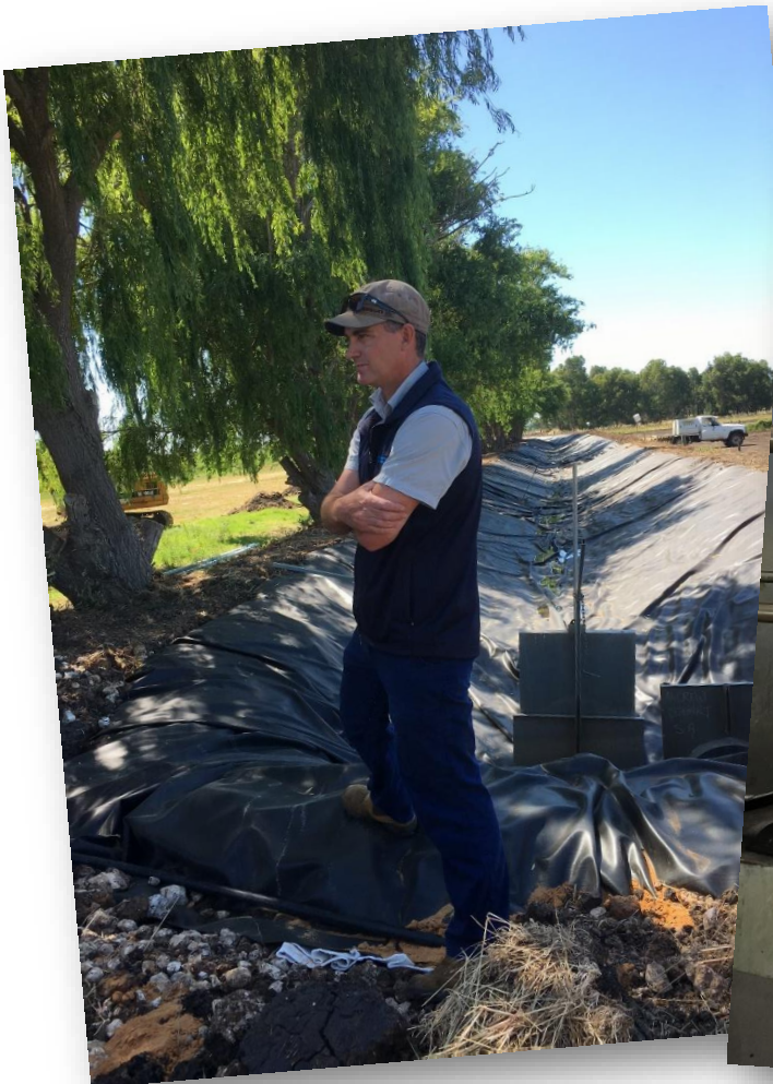
L: Michael Cutting lining an irrigation channel
